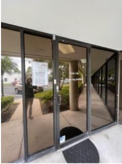
The front door as pictured here, is old, not up to current code, and doesn't lock fully even with the magnetic strip. The general public must be buzzed in and since we work with vulnerable Teens/Young Adults, the door has taken a lot of wear and tear and is not fully secure. If a person is not permitted into the building, there is a chance that with enough pulling action, they could open the door, creating a serious security risk for employees and clients.
