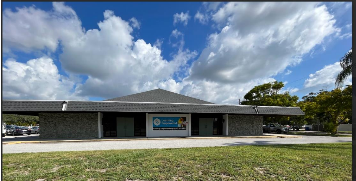
Proposed Family Engagement Center Project – facing 38 th Ave North and in front of childcare center and administrative/ mental health programming building
