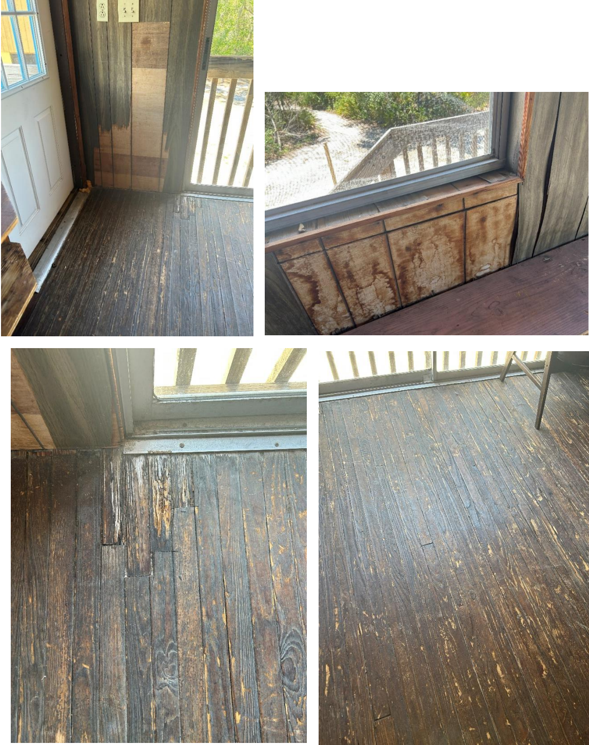
Figure 3. Examples of Existing Condition of Paneling and Flooring in Sleeping Cabins
